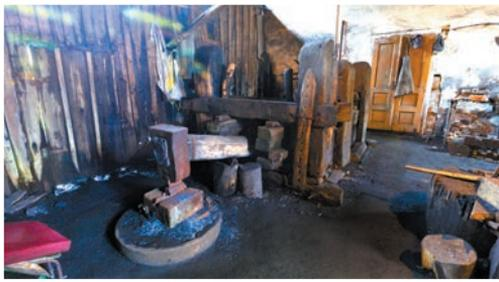
The forge in Lysychovo is the only functional water forge in Europe. The building is built on stone foundations. The walls of the west, north and south facades are lined with stones, and they are not plastered. The eastern wall of the facade is a wooden frame structure, and is plastered. The wall that divides the interior space into two parts, is lined using bricks. The roof is gabled with two gradients, currently lined with asbestos. A wooden manger is paced along the east wall.
